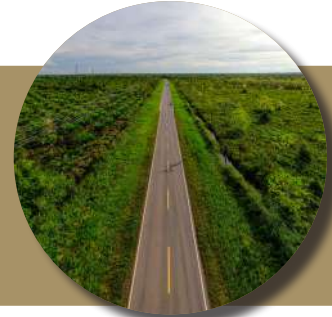
Jalan Road Infrastructure
